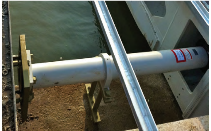
ACE oversized safety shock absorbers protect the lock gate by stopping 4,000-ton vessels.
