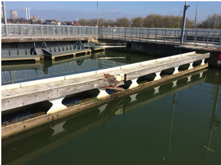
The ship lock's safety beam after a cargo ship had collided with it.
