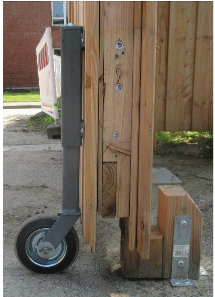
*Thanks to the springs, camp personnel have been able to roll the wooden gate with ease despite the uneven ground.*
